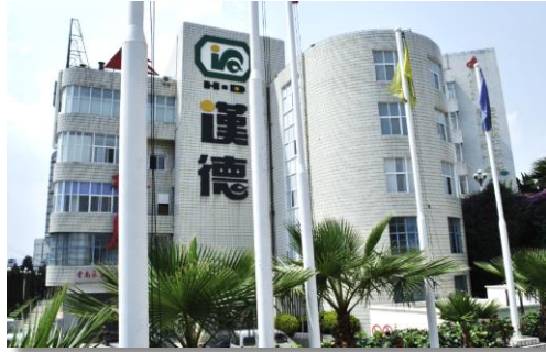
Plant A Overview (Founded in 1993)
